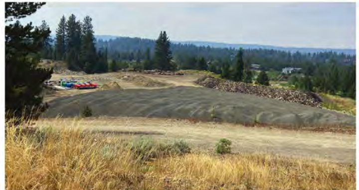
Existing Site Conditions
